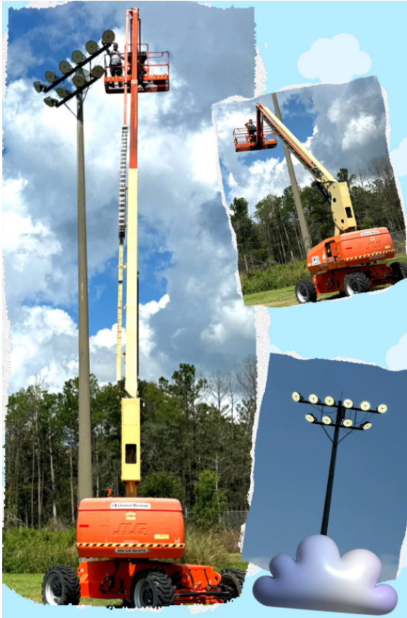
William Reed & Ron Johnson replacing LED light drivers
